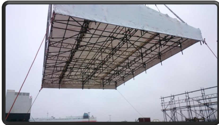
Liftable Roof Construction
